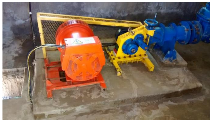
Figure 4: A micro-HEP turbine (blue, yellow) and generator (orange) located in Bario, Sarawak.
