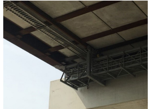
Fig. 3. Inspection platform used in practice.
