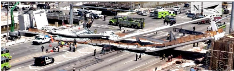
Fig. 2. Collapse scene of the pedestrian bridge.
