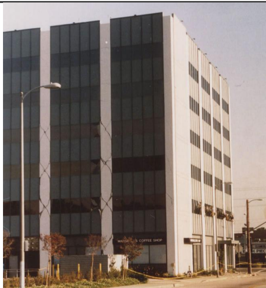
Figura 2.3 - Danni alle colonne del Barrington Medical Building (Faison et al., 2004).
