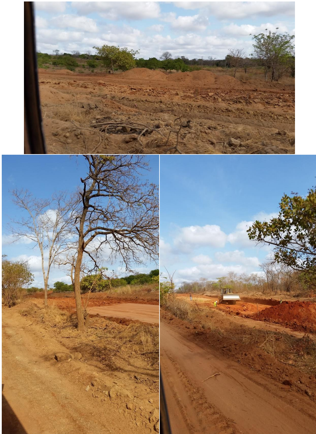
Figure 6.4 Examples of various stages of road construction work on Masasi-Songea Road
