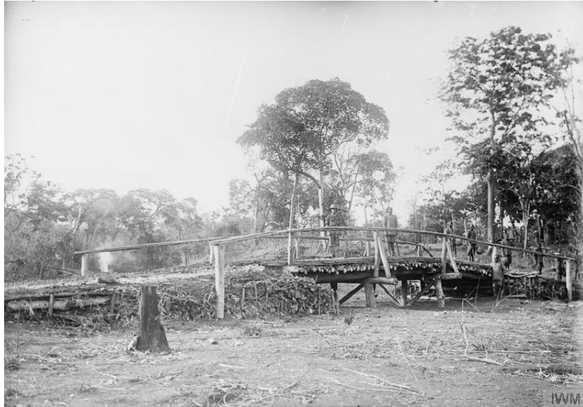
Figure 2.30 “All bridges were constructed with very few nails, dogs, etc. Supports were fixed in a position by the weight that was laid on afterwards. Near Ndanda. January 1918. Second Road Corps.” 267
