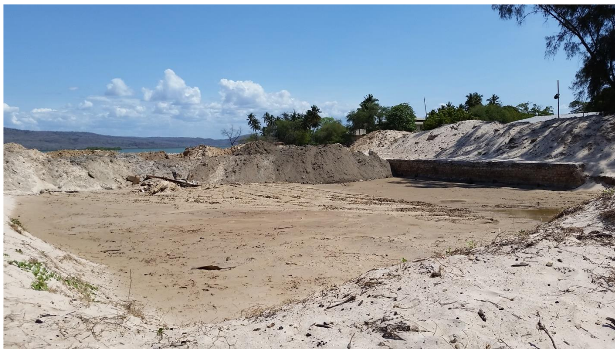
Figure 6.1 Construction Progress on Lindi Port, September 2015 18
