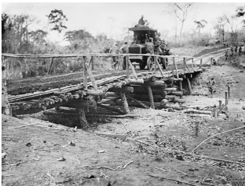
Figure 2.18 “Bridges built by No.1 section, 2 nd Road Corps, and constructed almost without nails or dogs. They were so built to take the heaviest loads. Nakin River, on the Kilwa Line. October 1917.” 236
