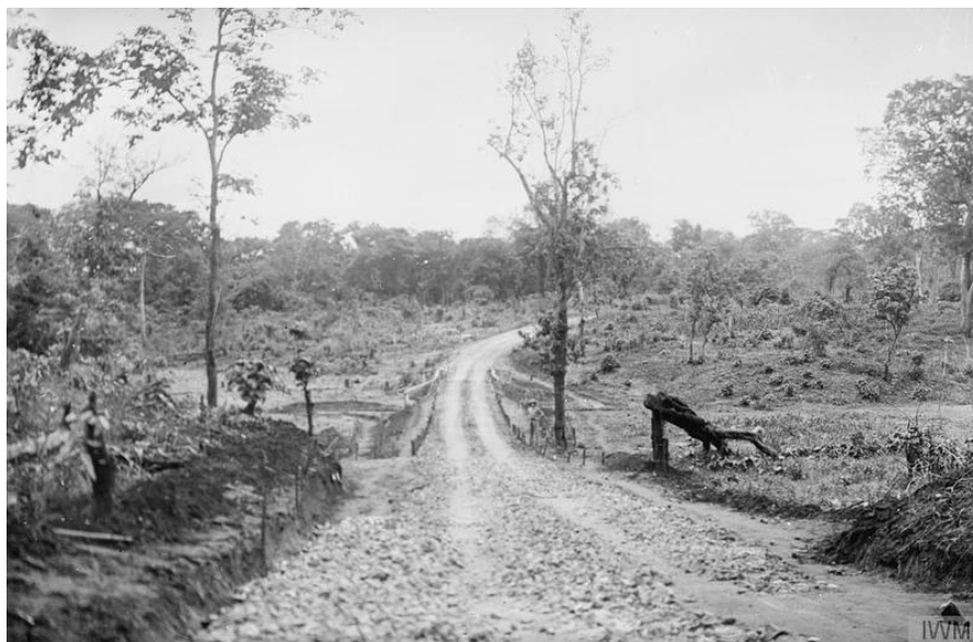
Figure 2.31 “Bridge and road made by 2 nd Road Corps, near Ndanda. December 1917.” 268
