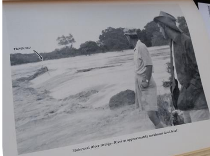
Figure 4.8 Destruction of the Muhuwezi River Bridge by Flood Waters, Tunduru, 1956 333
