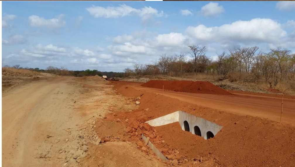
Figure 6.3 Construction progress on Masasi-Songea Road (outside Masasi)
