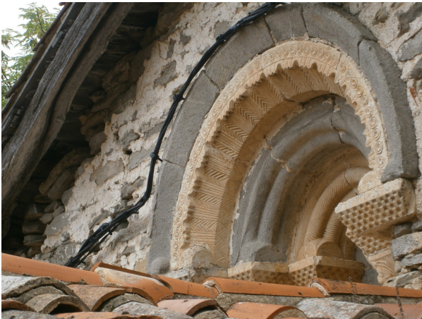
FIGURE 3. Church window of San Román de Arriano. Type 3 combination, white Paleocene limestones and dark bluish gray Upper Cretaceous limestones, with a strong colour contrast. Remains of lime that covered the entire facade, including the window.
