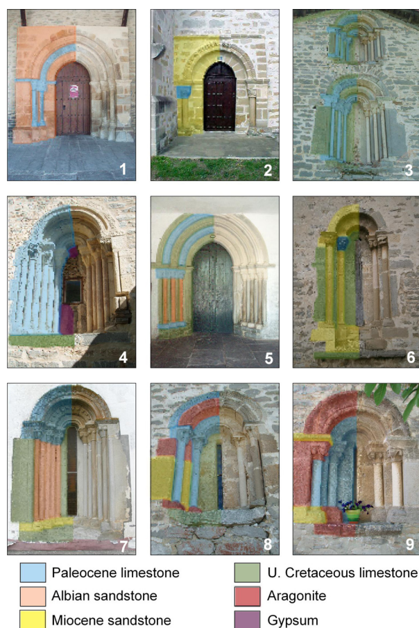
FIGURE 2. Lithological maps of the nine types of combinations in the most representative locations. Type 1: Respaldiza; Type 2: Bellojin; Type 3: Oyardo; Type 4: Délica; Type 5: Lezama; Type 6: Subijana-Morilla; Type 7: Belunza; Type 8: Ullibarri de Cuartango; and Type 9: Apricano.
