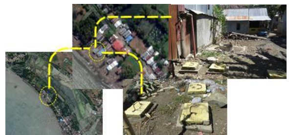
Figure 4. IPAL (Waste Water Disposal Installation)
