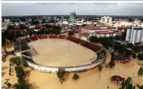
Figure 1. Sultan Muhammad V Stadium in Kota Bharu, the capital of the state of Kelantan, Malaysia, after Flood.
