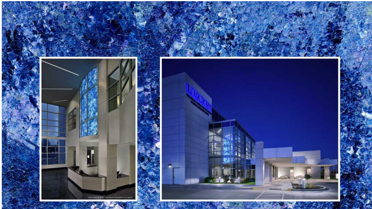
Lake Erie College of Osteopathic Medicine Wellness Center - Interior View Erie, PA
