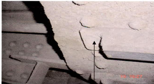
Remache instalado
