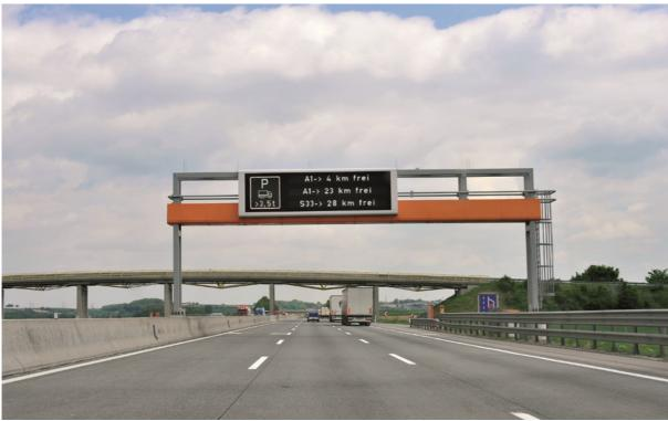
Figure 11 Intelligent truck parking. Image source/Copyright: ASFINAG
