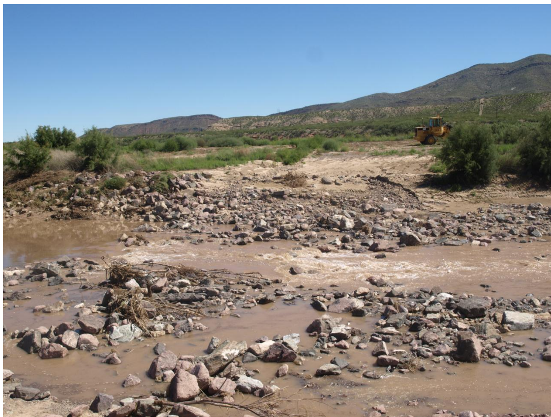
Photo 11: Temporary dike taken out by monsoons in 2013 (September 2013, AuBuchon)
