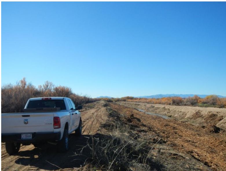
Photo 2: San Francisco Wasteway with maintenance mostly complete (November 2013)
