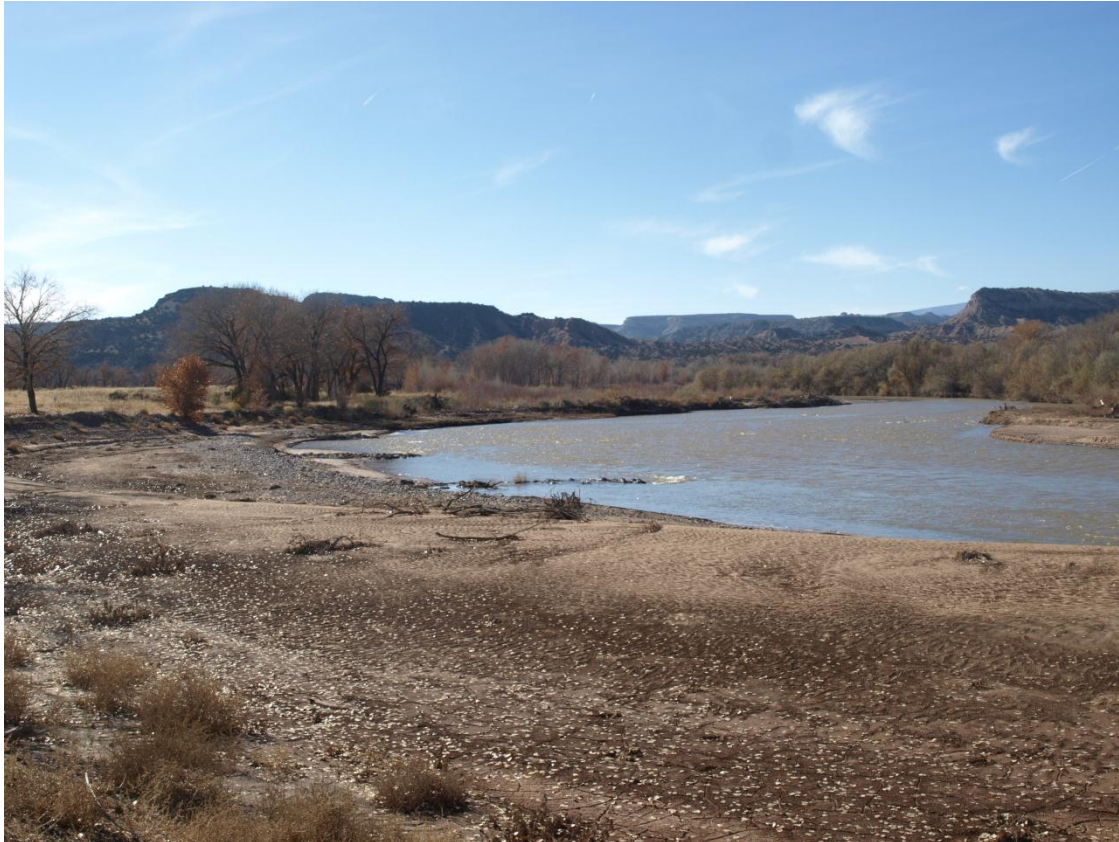
Photo 3: Constructed bendway weirs at San Ildefonso Priority Site (November 2013, AuBuchon)
