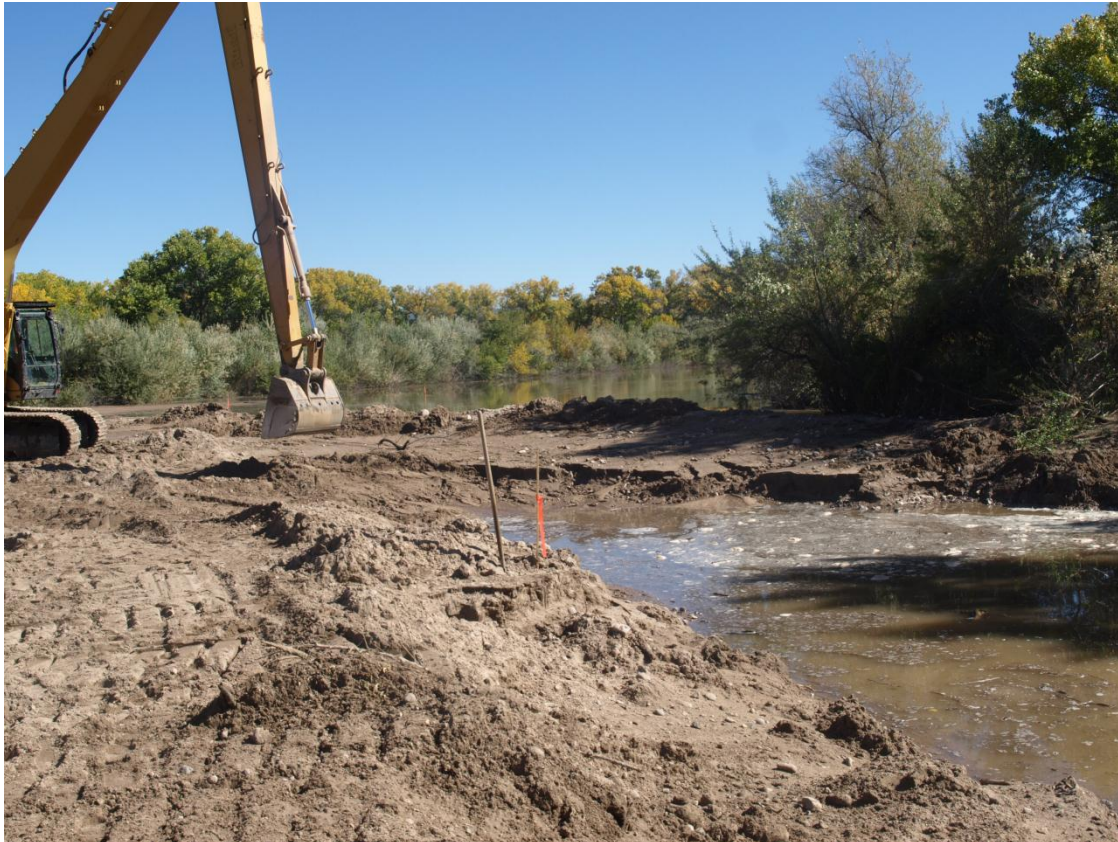
Photo 4: Construction of pilot channel at Peralta Arroyo (October 2013, AuBuchon)
