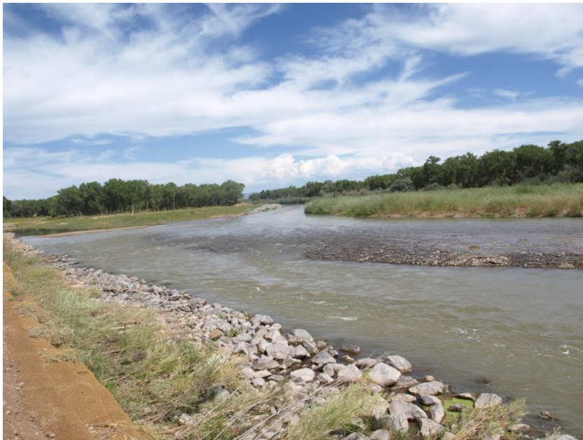
Figure 9: Looking upstream after completion of RM 223.9 Site
