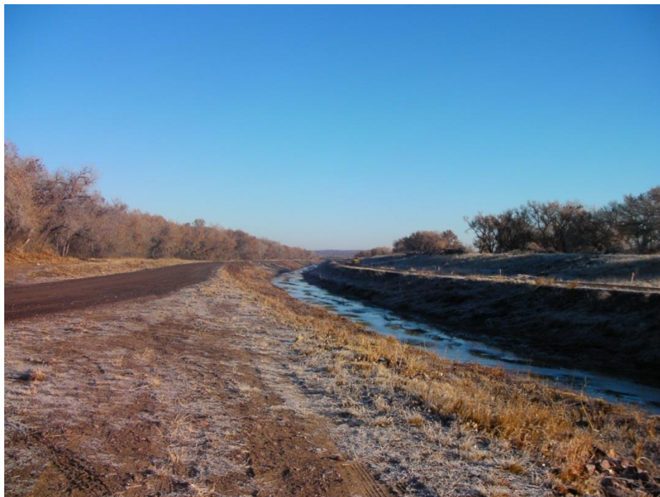
Figure 5: LFCC mowed areas at Otero Bridge (Jan 2015)
