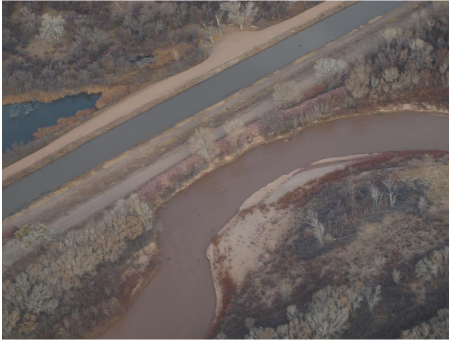
Figure 13: Fort Craig Bend, pump site, and LFCC (December 2014, Aubuchon)
