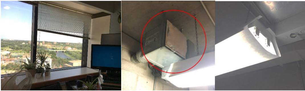
Figure 3. Examples of obstructions of building controls and occupants' adaptations to improve their comfort
