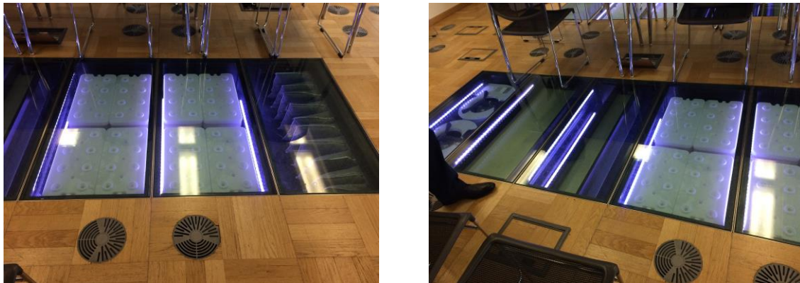
Figure 95: Example of PCMs integrated into an Air Handling Unit. South Bank University. London, K. Source: author.
