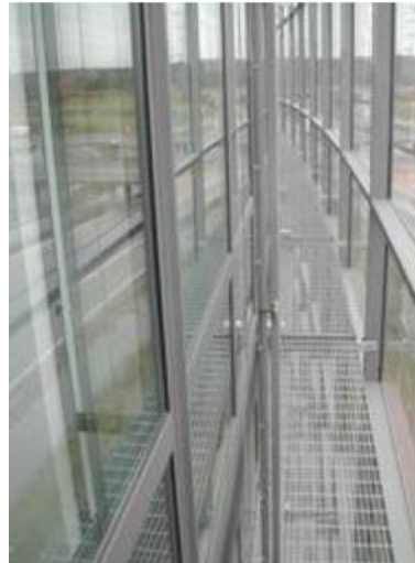
Figure 93: Glazed building with double skin façade.
