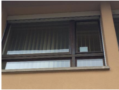
Figure 49: Window opening details of Bulach school. Source: author.
