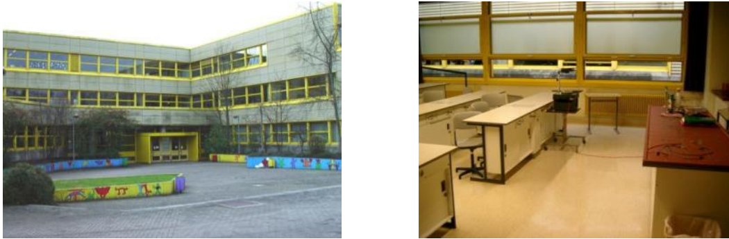
Figure 30: Example of a school building from the 1970s in Karlsruhe: Sophie Scholl Realschule Karlsruhe. Source: HGW (2016).
