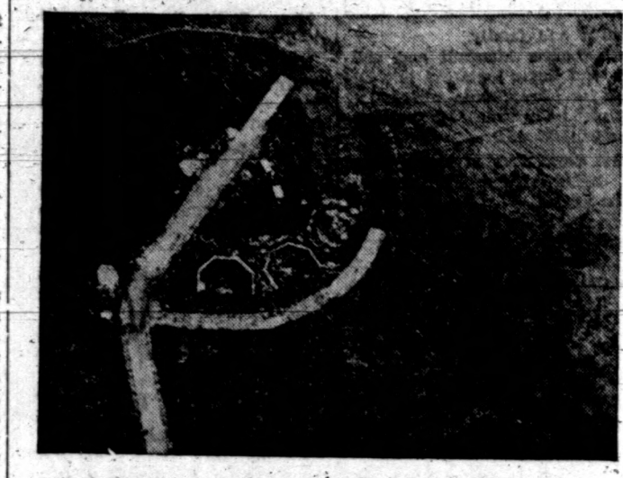
Aerial view of valuable Solomon Island airport, captured by U. S. Marines shortly after they launched their attack upon Guadalcanal, which has been the objective of numerous attacks staged by Japanese. Note the U-shaped revetments being constructed for protection against strafing.
