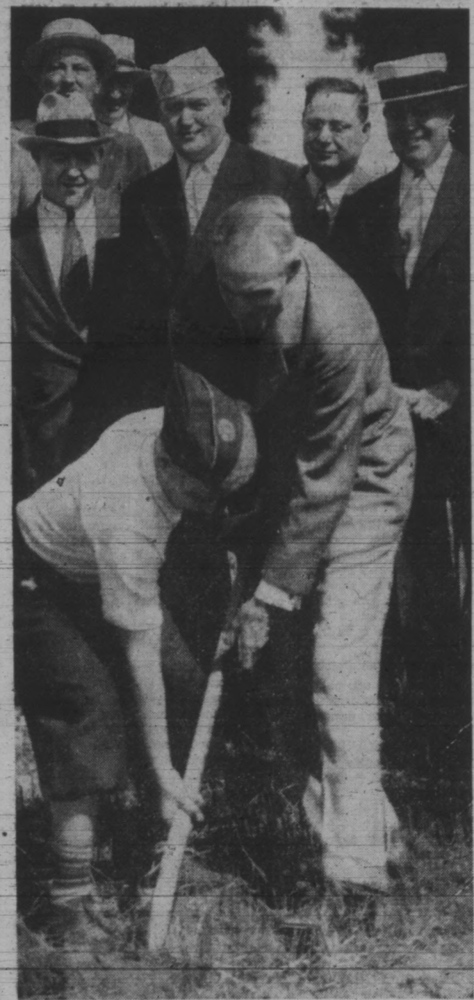
• DONALD ADDY helps HENRY FORD break ground for the new veterans' hospital to be built in Dearborn.
