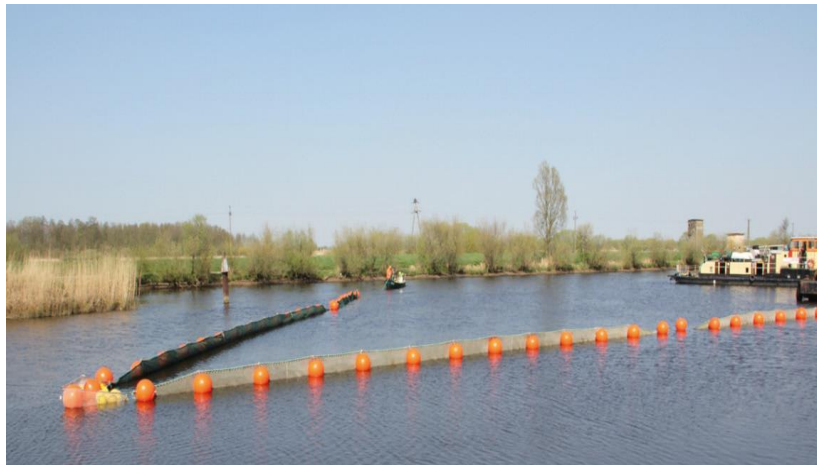
Figure 9: The boom in operation
