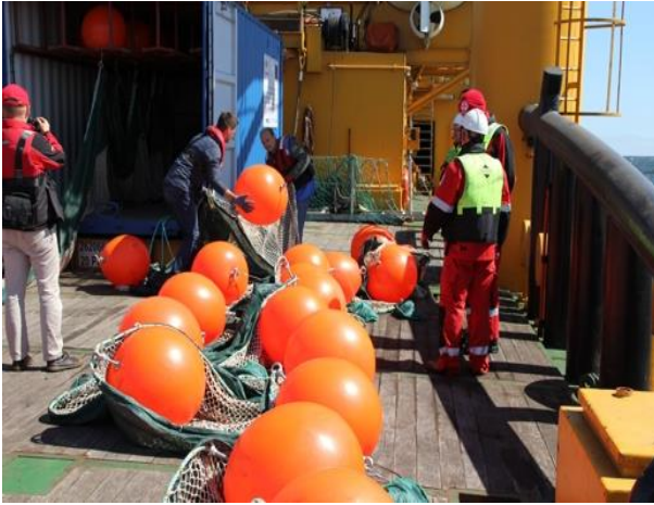
Figure 10: The boom is discharged from container
