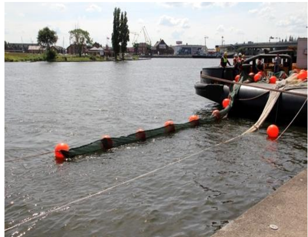
Figure 13: The boom discharging
