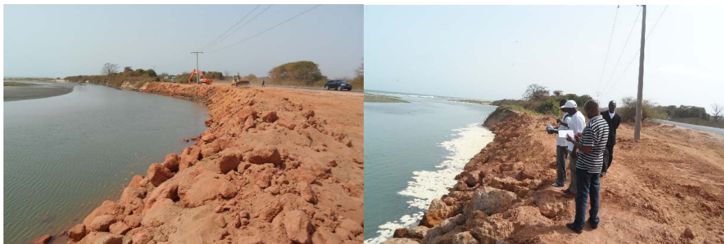
Figure 8: Lateritic rocks used as coastal construction materials at Tanji bridge
