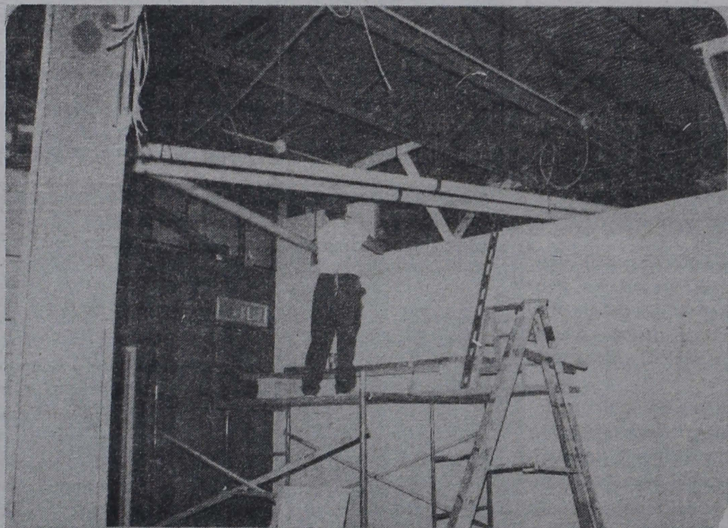
Construction for the Wisner Move has already begun.
