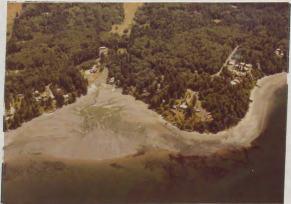
FIGURE 21. Oblique aerial photograph showing the wave-cut platform at Dickenson Point. View is toward the southwest.
