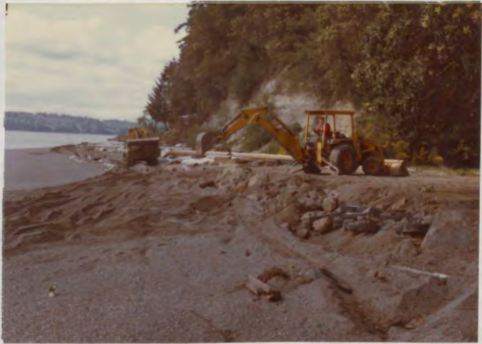
FIGURE 18a. View north showing the westward readjustment of boulders and tires along the spit at Burfoot County Park. Photo taken 5/12/82.
