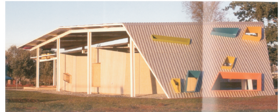
Figure 063. The roof plane serves as a multi-functional object, one that defines spaces, plays with light and views and allows interaction
