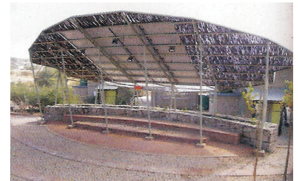
Fig 085. Solar Panels incorporated into an overhead plane
