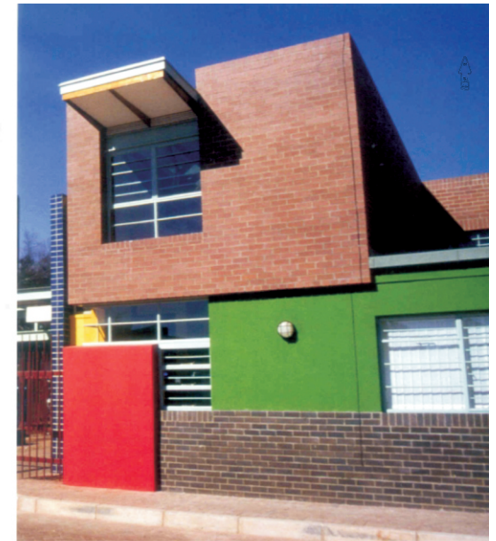
Figure 041. Photo of Yeoville Clinic
