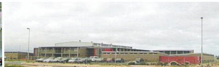
Fig 060. School building on approach
