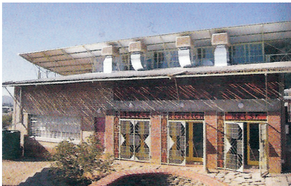
Fig 083. Shaded Northern Facade
