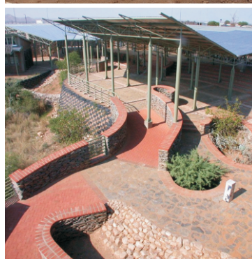
Fig 078. Overlooking the Multi-Use Area
