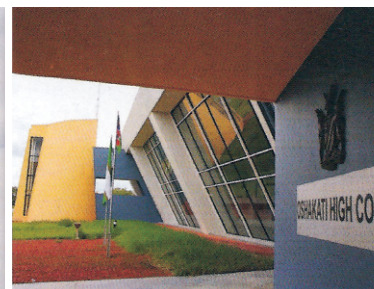
Figure 045. Windows slanted at 30° to limit solar insolation
