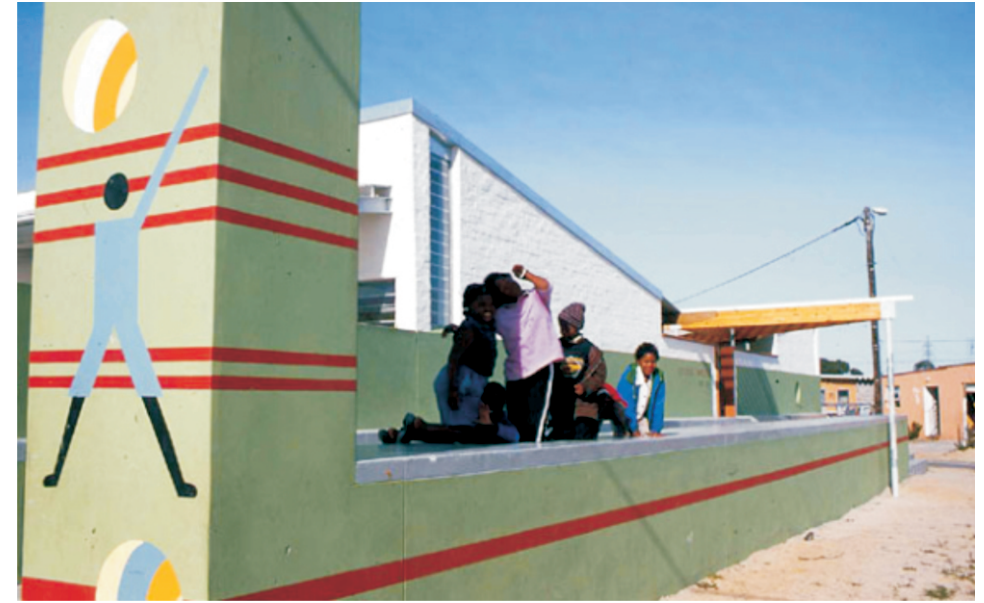
Figure 062. Street facade of Delft Day Care Centre
