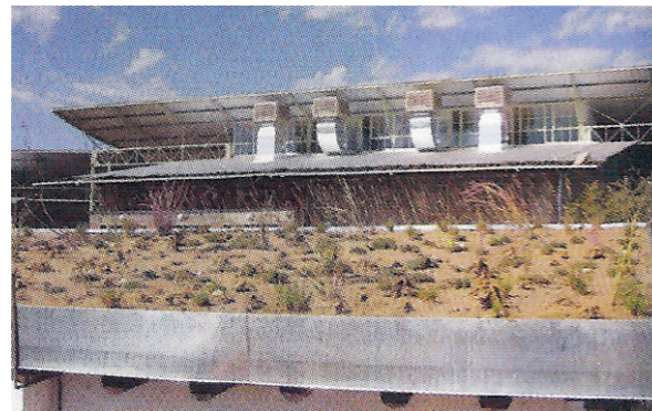
Fig 084. Roof top planting acts as insulation
