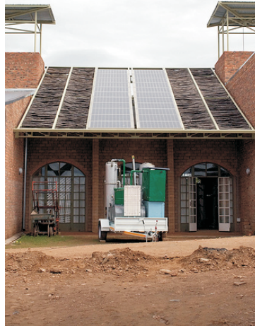
Fig 076. Solar Panels provide power to the development
