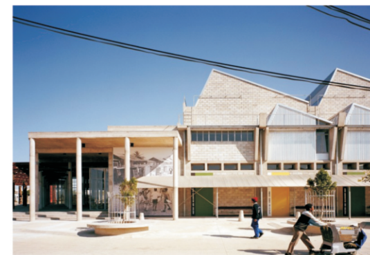
Figure 033. Photograph of the Eastern Facade. Simple tectonics and the use of materials common to the area integrates the
