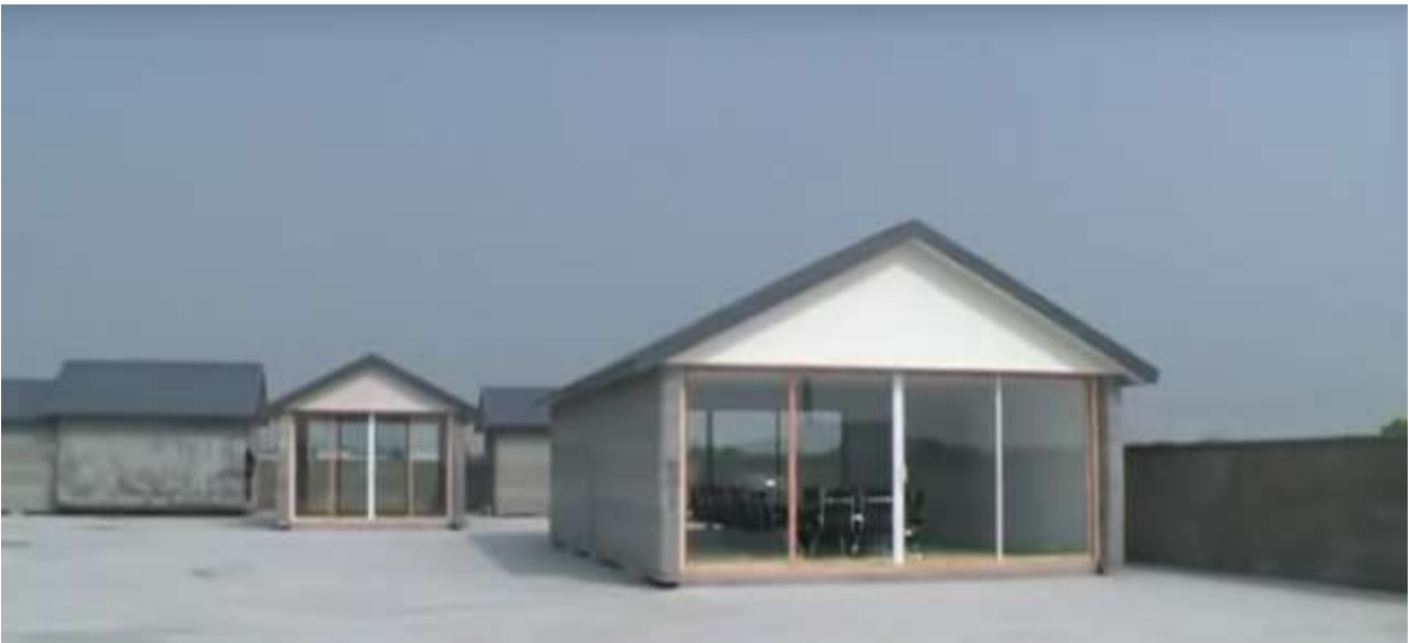
Figure 3.6.4: 10 houses 3D printed in 24 hours
