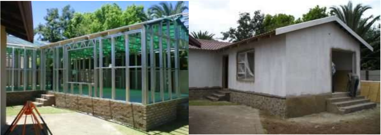
Figure 3.6.6: Before and after pictures of a residential light steel project
