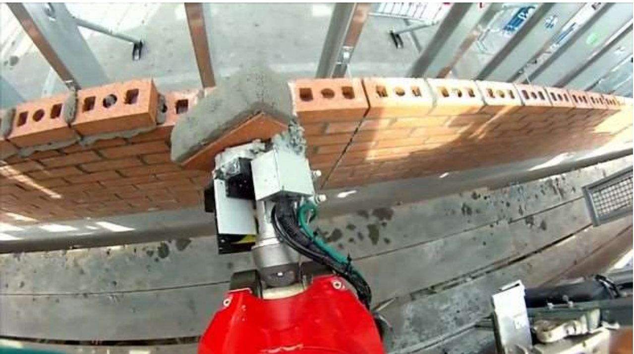
Figure 3.6.5: Semi-automated mason construction robotics
