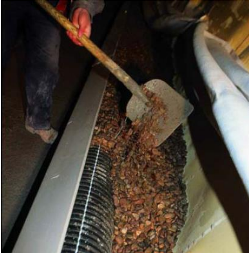
Backfilling of Sika Drainage angle with gravel -> high drainage capacity
