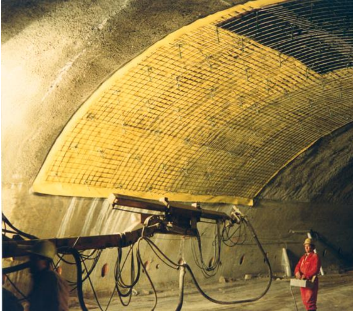
Inner Shotcrete onto Membrane
