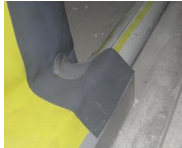
Connection with membrane by spot-welding
