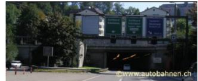
Figure 4: North portal of Reussport Tunnel.
