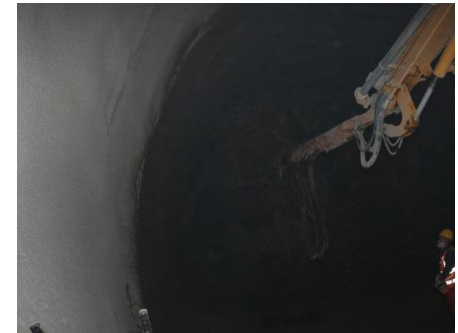
Concrete spraying
