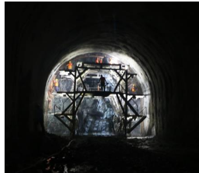
Grid arch arrangement
