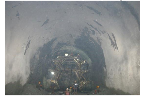
Overall situation of support
