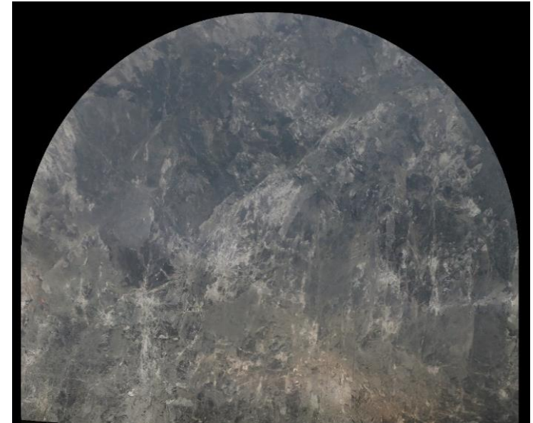
Surrounding rock condition of excavation face at X2K0+240
