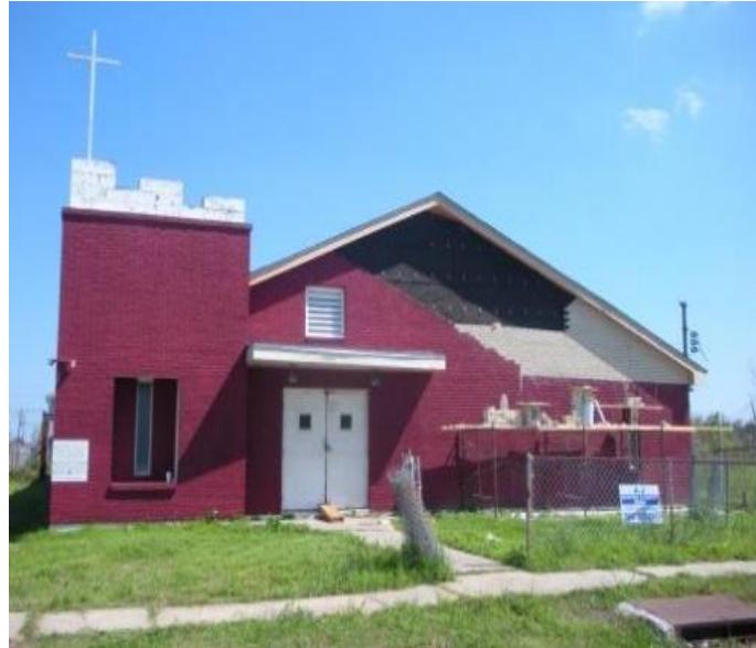
Figure 8- Battleground Baptist Church being repaired post-Hurricane Katrina
