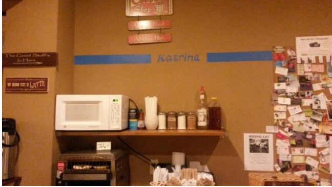
On a wall in a café, a painted blue line denotes flood depth level inside of the building
