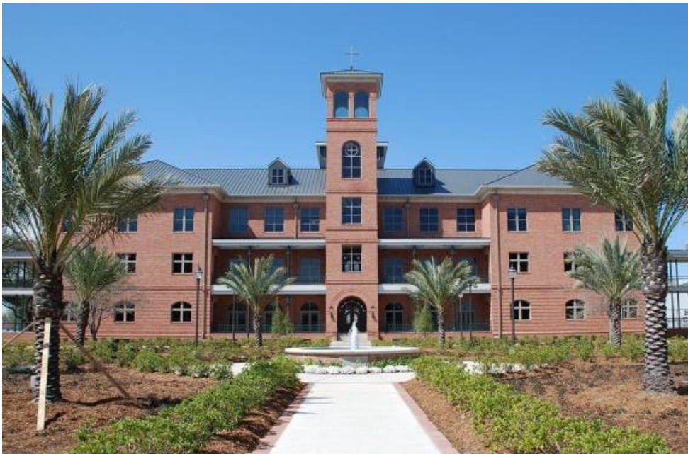
Relocated (from the Lower Ninth Ward to the Gentilly neighborhood) and rebuilt
