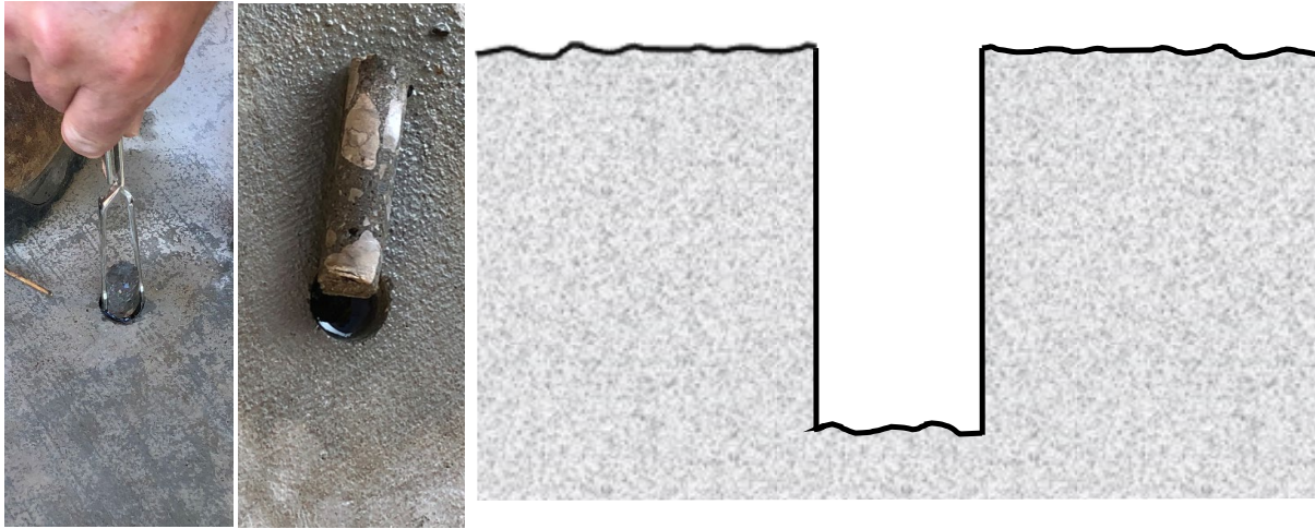
Figure 3 Remove core and ensure the hole is cleaned out.
