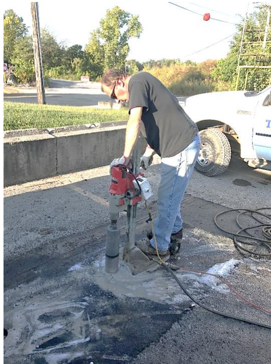
Figure 1 Cutting Polymer Asphalt cores
