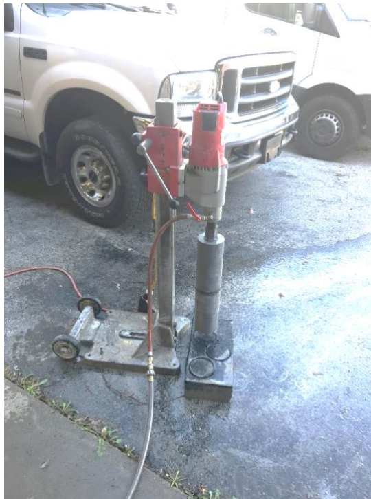
Figure 2 Cutting Cores from Concrete Cap Blocks
