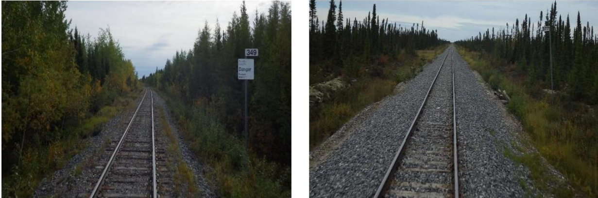
Figure 7. Photos of milepost 349 (left) and milepost 377 (right) showing population of trees and no surface water ponded close to the embankment shoulders.
