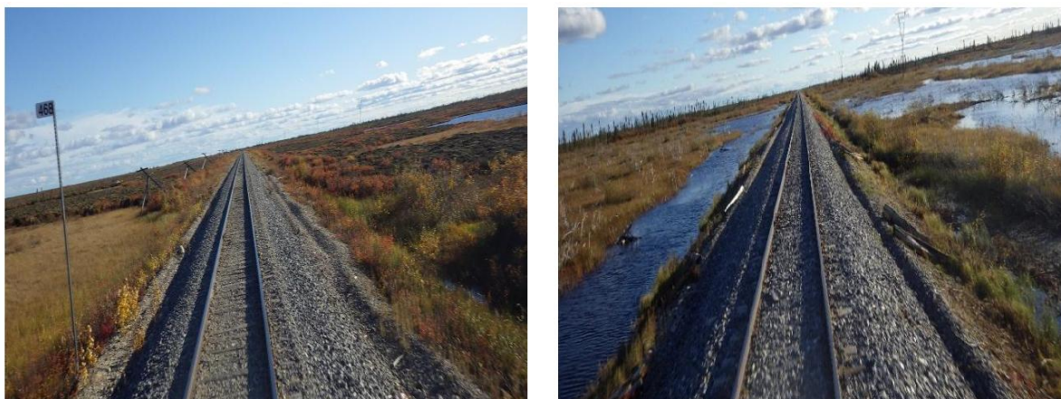
Figure 6. Photos of milepost 468 (left) and milepost 448 (right) showing no tree cover and ponded water close to embankment shoulders.
