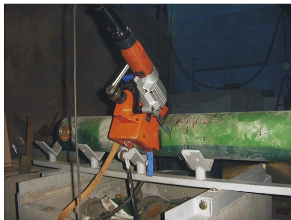
Figure 5. Cutting of the first cooling systems pipe
