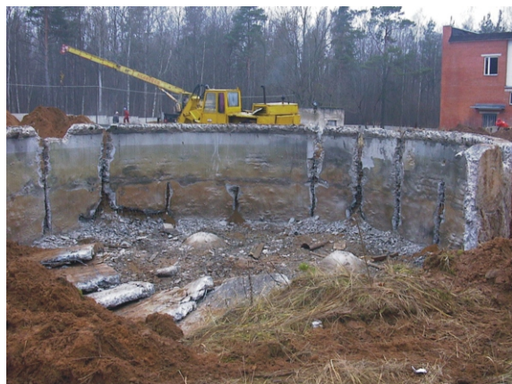
Figure 4. Dismantling of 400 m 3 tank in the SRR yard
