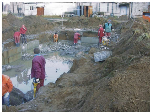
Figure 3. Dismantling of second cooling system pumps basement
