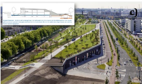
Fig. 6. Examples of coastal protection in the Netherlands. 6.a. Storm surge barrier Maeslantkering, as a historical solution, part of the Delta works. 6.b. Integrated dunes and parking at Katwijk; 6.c. Dakpark: integrated roof-top park and dike at Rotterdam; 6.d. Integrated flood walls, sand nourishment, and dikes at Scheveningen.
