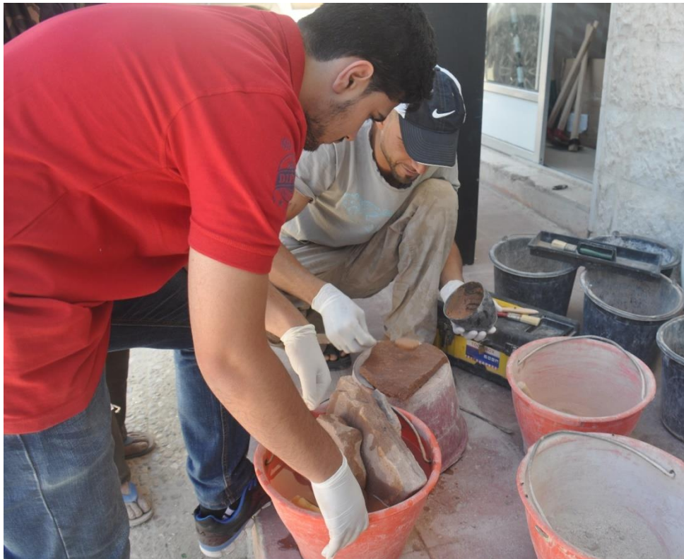
Picture 5: One of the Hashemite students, Ahmad Daffar, is learning how to prepare lime mortar with Sela trainer, Ahmad Mowasa. (Photo credit: Halemah Nawafleh)
