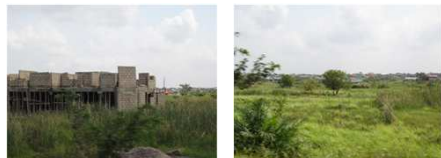
Figure 1a and 1b. Urbanising land: Buildings in various stages of completion
