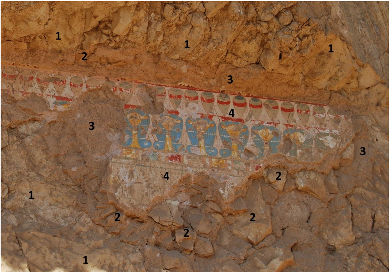
Image 16 – Western wall of the northern end of transverse hall. Stages of \text{z}^{\text{cc}} . (1) Natural rock. (2) Primary stage of \text{z}^{\text{cc}} (coarse plaster with heavy inclusions of limestone flakes). (3) Secondary stage of \text{z}^{\text{cc}} (coarse plaster). (4) Fine gypsum plaster with coloured decoration. Photograph by Heidi Kontkanen, 2011.
