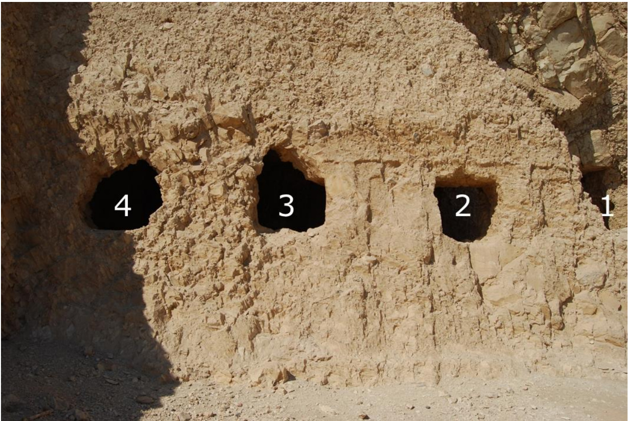
Image 15 – The remaining façade of TT 71 on the southern side of the entrance. Notice the carved stone between window 1 on the right (mostly destroyed when the roof of the transverse hall collapsed) and window 3. This stonework is missing between window 3 and 4 possibly due to an expansion of the façade and/or the courtyard. Photograph by Heidi Kontkanen, 2011.
