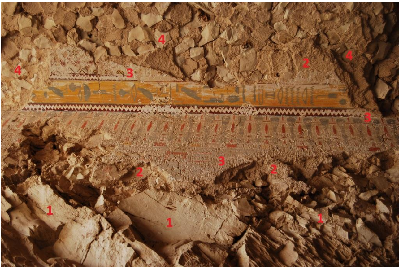
Image 6 – South wall and ceiling of the axial hall showing the natural rockface (1), layers of plaster (2), the coloured decoration (3), and plaster inset with limestone chips (4). Photograph by Hanne Siegmeier, 2011.
