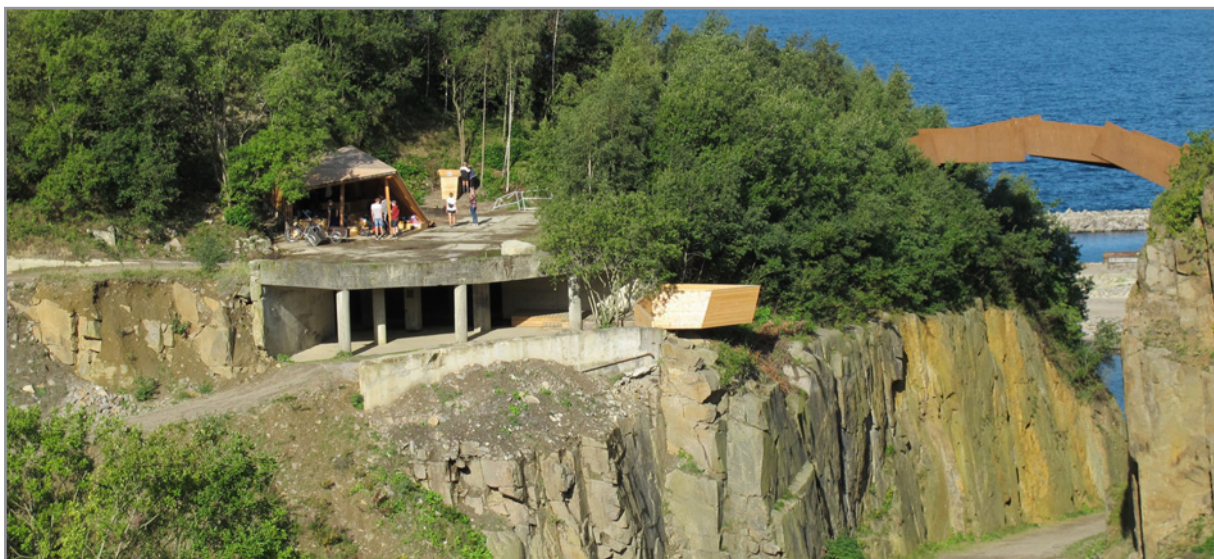
Figure 8: The new shelter and viewing point on top of the derelict granite crushing plant. Photo: Vivi Granby.
