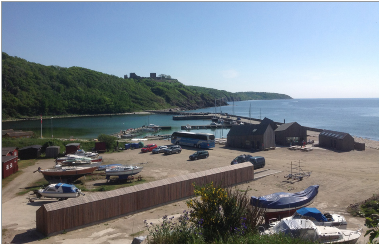
Figure 4: View of Hammer harbour with the new kayak shed and the cluster of new facilities; in the background, the ruins of the medieval castle, Hammershus.
