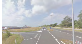
OSKARFREDVÆJ The big road (Oskarfredvej) that is going all the way to Randers, is a major barrier to the connection between Nykøbing S. and Nordstrand.
