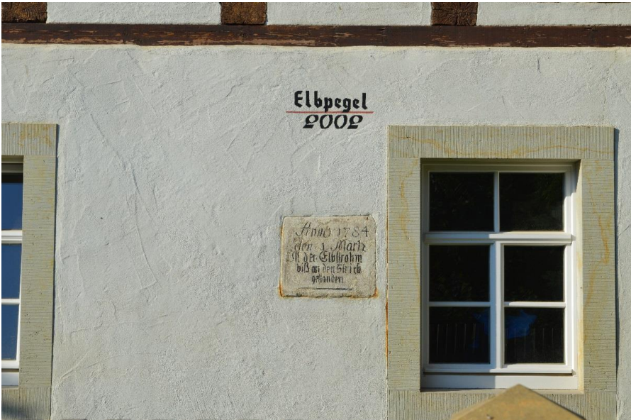
Figure 15. Watermarks in Gohlis, Dresden. The above watermark is from the 2002 floods, and the faded, older one, is from the 1784 floods. Photo: Kristoffer Albris, 2015.
