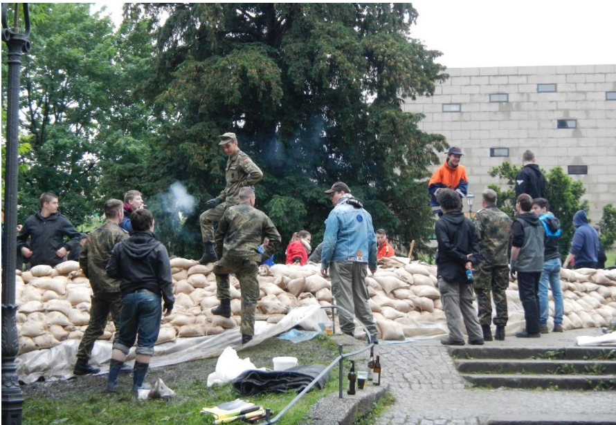
Figure 19. Work at the sandbag dikes by the Bärenzwinger Student Clubhouse. Top: unloading of sand and a group of volunteers waiting to fill bags. Bottom: Bundeswehr and volunteers coordinating in cooperation with one another. Photo used with permission.
