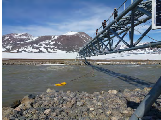
Figure 45: Discharge measurements are performed along the hoist trolley. Q.liner is attached to the steel wire.
