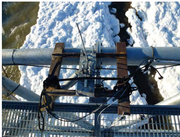
Figure 43: Metal frame for installation of OBS, diver and conductivity sensor
