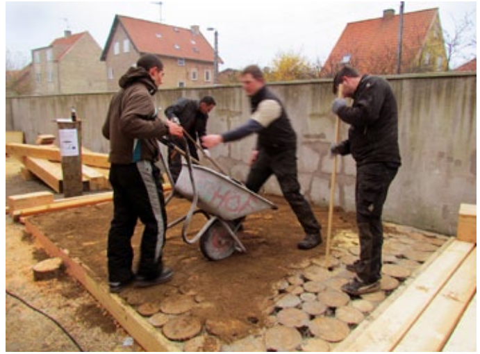
FIGURE 2. Wood is being assembled into terrace floors.
