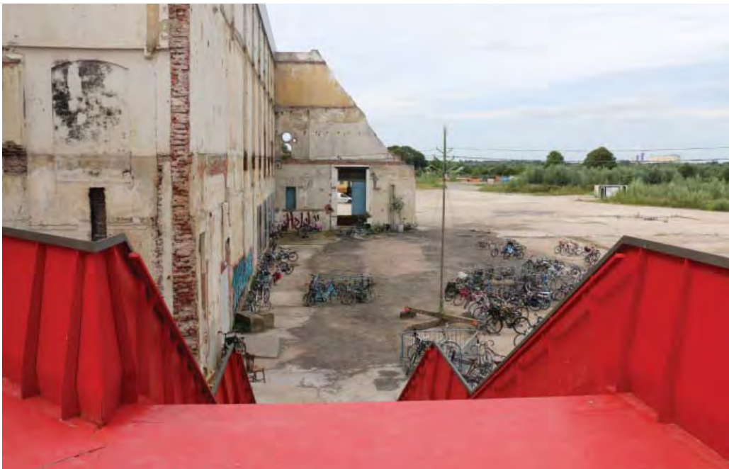
^ 12.08.2015_The office of the new site management team is built into the lower part of the sieve building
