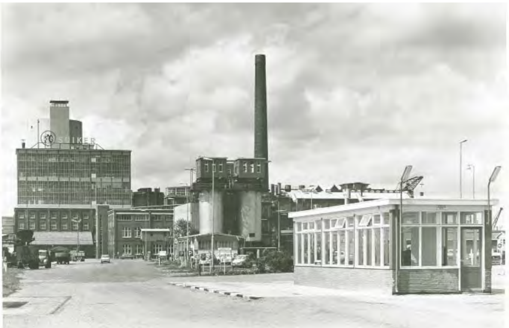
Friesch-Groningsche Beet Sugar Cooperative in 1963 . Factory seen from the main entrance (Heemskerckstraat), in the foreground the weighbridge building (Source: RHC Groninger Archieven)
