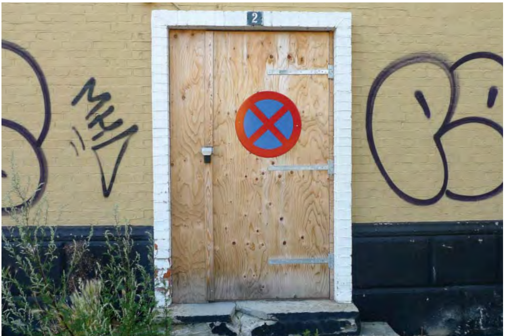
08.07.2013_The buildings on Smedestræde are sealed off to prevent break-ins.
