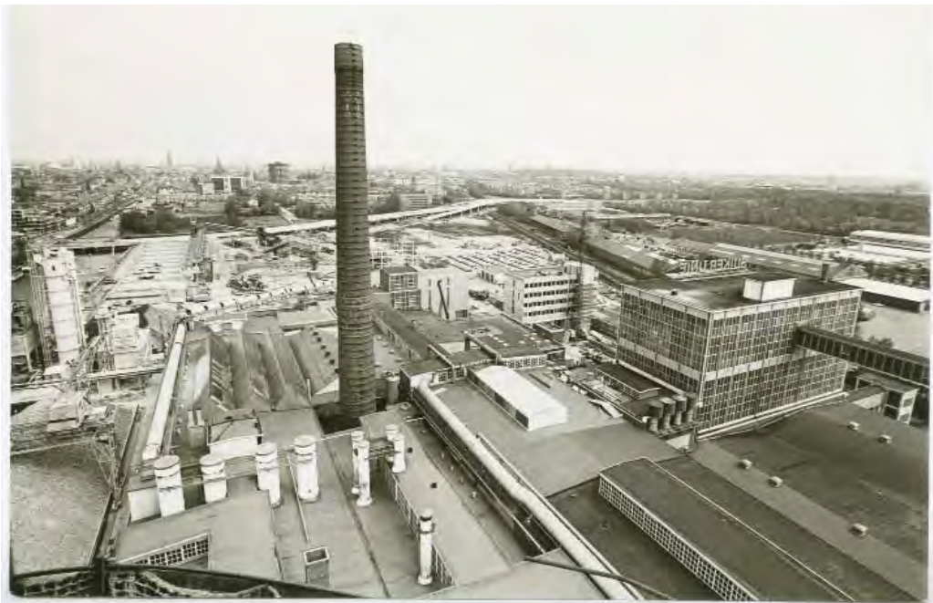
Overview of the Suiker Unie factory complex towards east in 1975 (Source: RHC Groninger Archieven)
