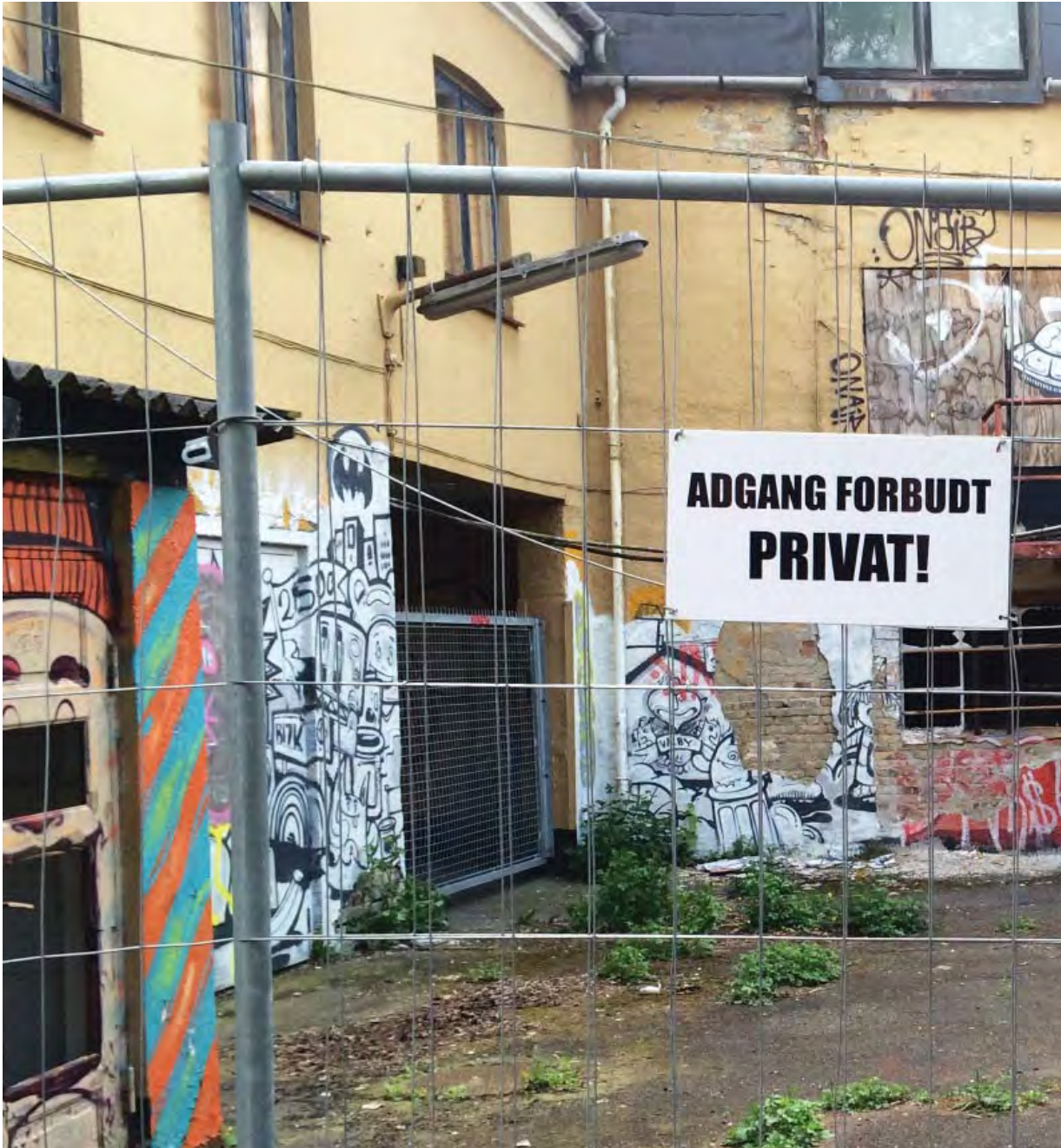
14.05.2016. 'No Entry - PRIVATE!' signs and wire fence surrounding the decaying buildings at Smedestræde 2 in Valby. But what kind of 'private'? The property is owned by the Copenhagen Municipality. The sign refers to conventions in terms of behaviour: Private here reinforces the 'keep off'- message.
