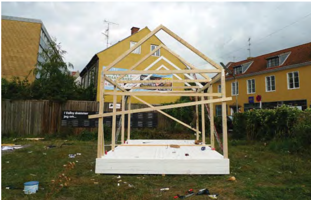
29.08.2013_The Valby Pavilion in construction in August 2013
