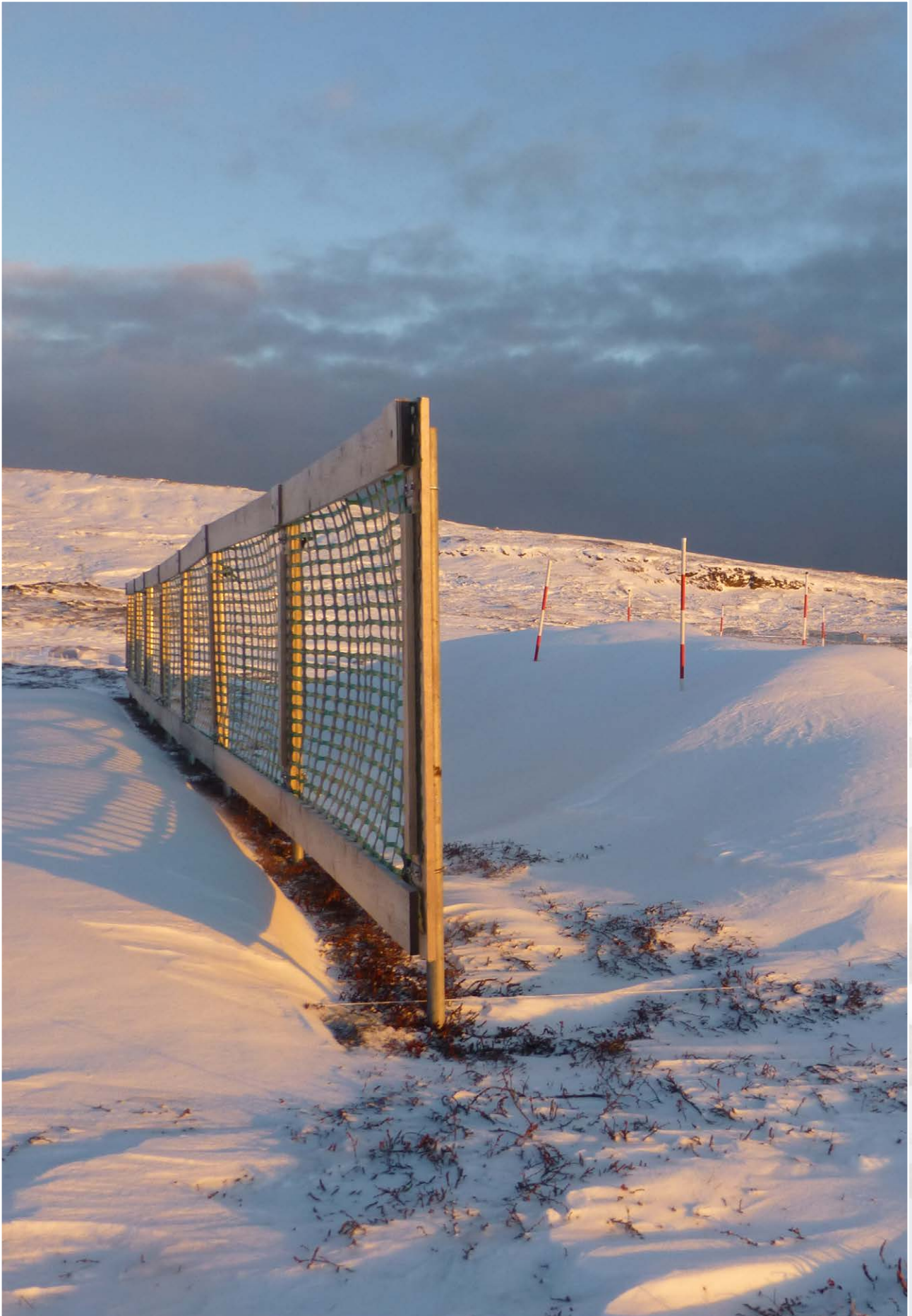
Snow drift building up on the lee side of the snow fence (photo: Charlotte Sigsgaard).
