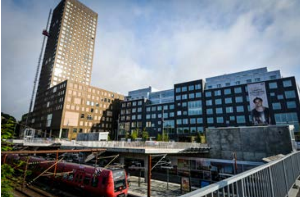
Fig. 8 Carlsberg's largest new-built complex is a quite generic structure. It does not adopt significantly to the industrial architecture nor the activities of the people that had used Carlsberg after the financial crisis. Photograph from 2016 Svend Rossen/UCC.
