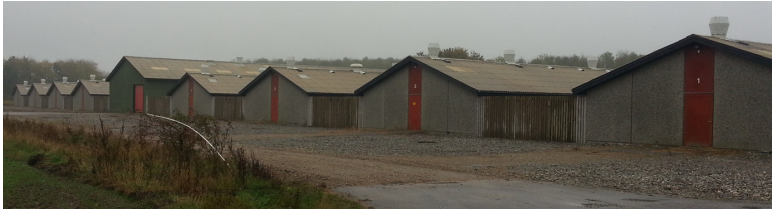
Fig. 2. The wooden walls separating shielding the space between the sections. The photo is taken on the East-side of the station.
