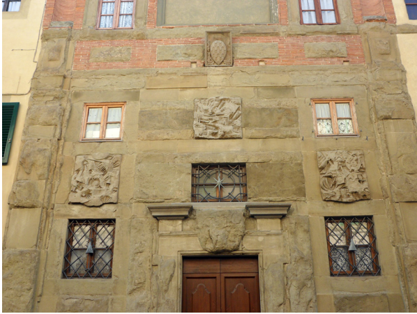
Figure 10. Federico Zuccari's house. 1578. Florence (photo: Roberto di Ferdinando).
