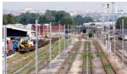
Fig. 55. Existing rail yard at Aygalades (photo: Eric Lion for the Leclercq team)
