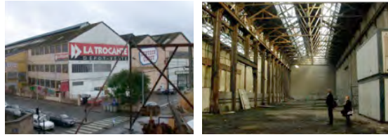
Fig. 4-5. The Nefs at the Chantiers site as found and under construction, showing its basic metal structure (source: conference Chemetoff 2010)
