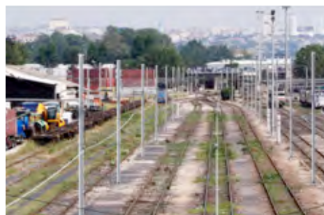
Fig. 51. Existing rail yard at Ayalalades (photo: Eric Lion for Leclercq team)
