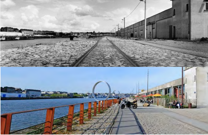
Fig. l. Quai des Antilles before and after transformation (top photo: Arnauld Duboys Fresney for Samoa; bottom photo: Vincent Jacques for Samoa)
