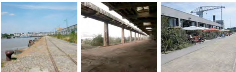
Fig. 8-9. The Banana Hangar site as found and under construction, showing its basic concrete structure (source: conference Chemetoff 2010)
