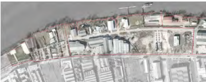
Fig. 16. Aerial photo of the Angélique site with its harbour wasteland on the riverbank (outlined) and the adjacent industrial plots, 2009 (source: Desvigne 2009)
