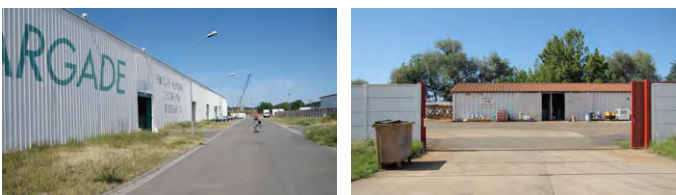
Fig. 17-18. Existing buildings on the riverbank, 2012 (photos: L. Diedrich)
