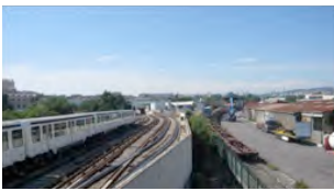
Fig. 114. Rail yard at Aygalades 2012 (photo: L. Diedrich)
