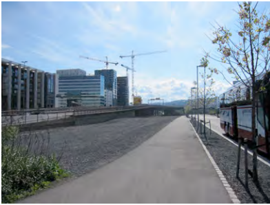
Fig. 16. Bjørvika Bay's waterfront with the construction site of the Bar Code, 2010 (photo: L. Diedrich)
