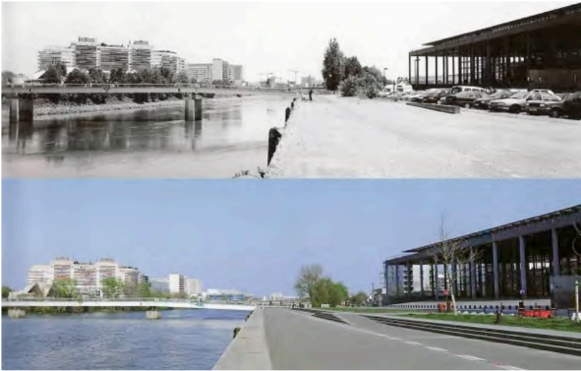
Fig. n. Quai François Mitterrand in front of the new Tribunal before and after transformation (top photo: Arnauld Duboys Fresney for Samoa; bottom photo: Vincent Jacques for Samoa)
