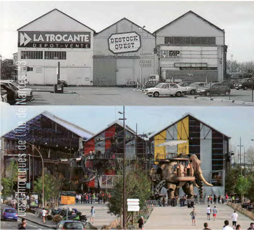
Fig. m. Les Chantiers before and after transformation (top photo: Arnauld Duboys Fresney for Samoa; bottom photo: Vincent Jacques for Samoa)
