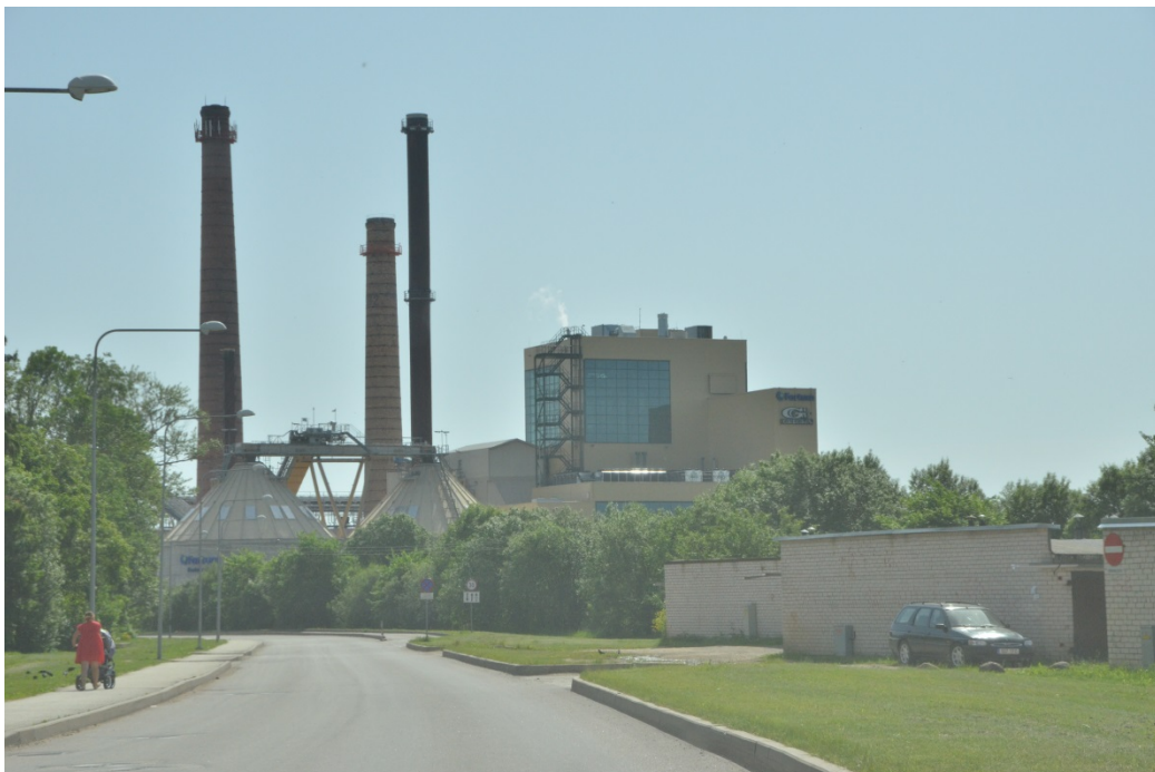
Figure 30: New combined heat-power-plant (CHP), Tartu (field work, June 2014)
