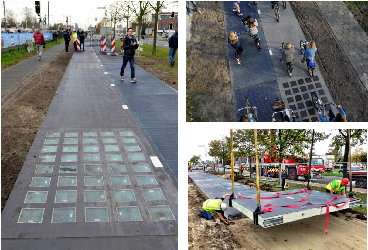
Figure 5.15: Solar cells on bicycle lanes
