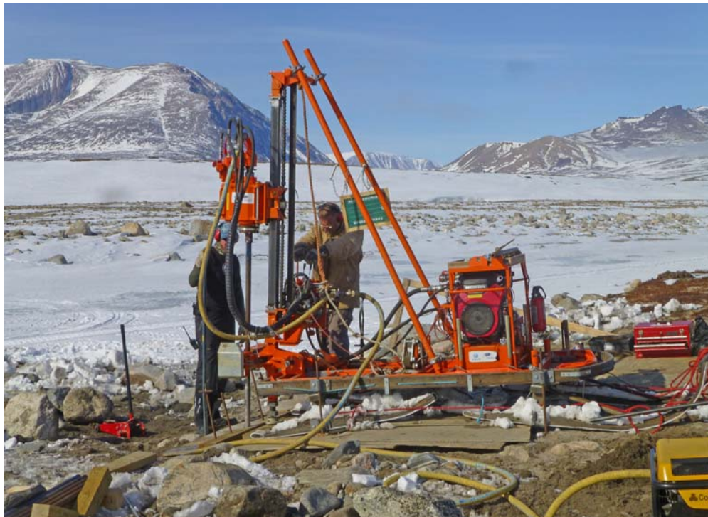
Figure 6.44 Drilling boreholes for the anchor points. Photo: Mikkel Tamstorf.
