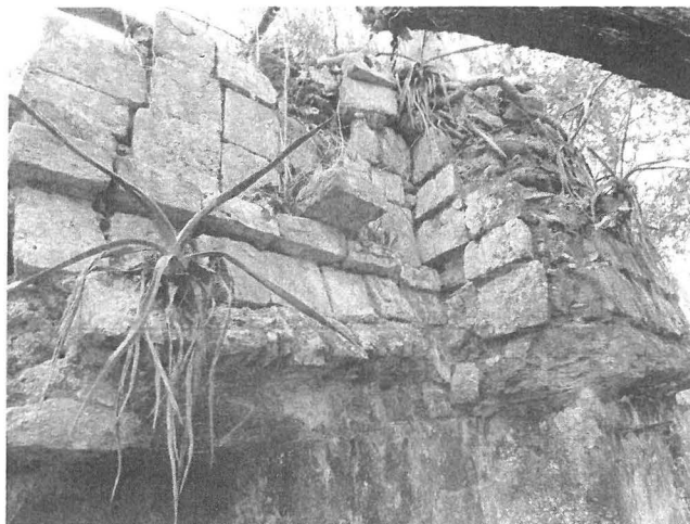
Fig. 12. Upper façade, western part of main façade, Structure 2. Photo: Stephan Merk, 2015.
