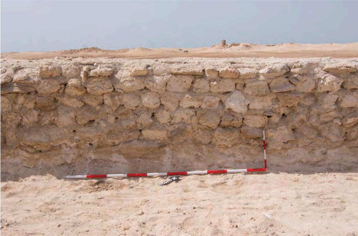
Figure 5.4: Condition of the outer shell of the Outer Town Wall before conservation. The brittle beachstone is extremely eroded. Hard cement mortar can be seen in horizontal layers. (YE-0229)
