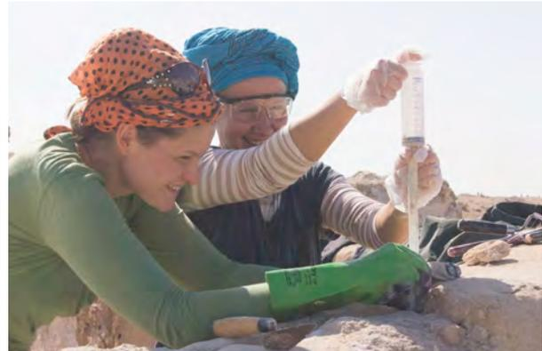
Figure 4.12: Restorers filling voids in the wall with liquid mix. (XF-0213)
