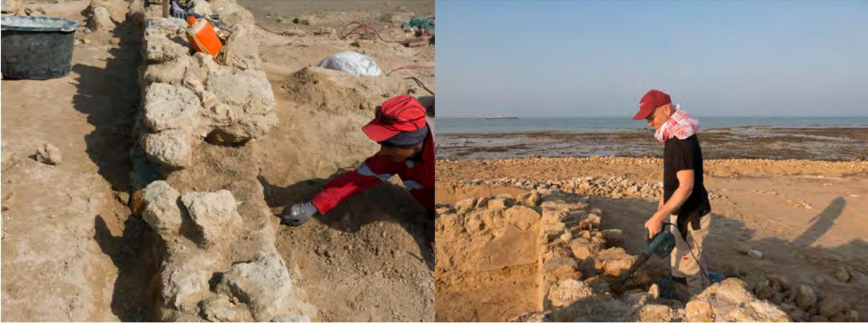
Figure 7.14: Dust, dirt and loose stones and mortar were removed with trowel and hand brush; eroded joints were scraped and cleaned with a blower before being repointed. (WE-0013 & WE-0040)
