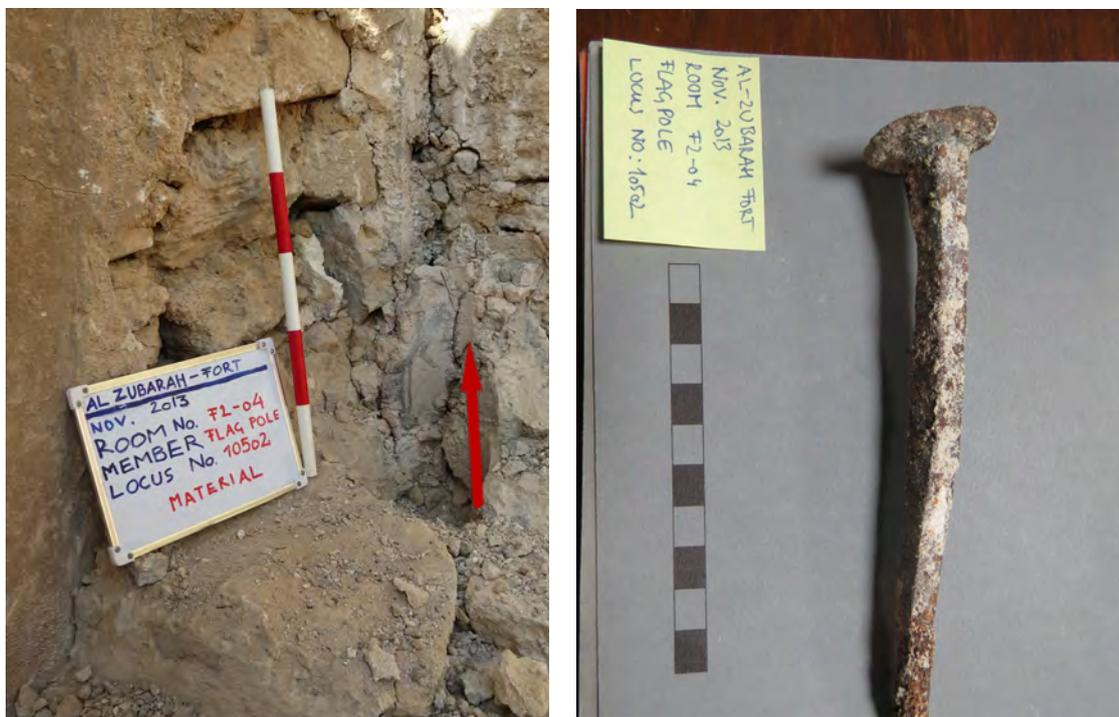
Figure 6.9: Left (ZUTE-0061): Masonry block for the flag pole during its demolition. The cement-based plaster shows a circular void with the impression of the texture of a wooden trunk (arrow). Right (ZUTE-0084): Hand-forged nail found in the masonry of the flag pole base. Similar nails were found in the dhow mast.
