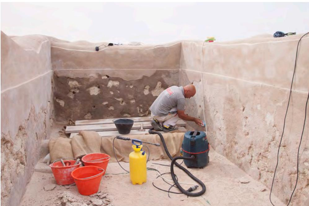
Figure 3.22: Preparation of walls in Space 3005 for void repair. Detached plaster were removed. (DF-0378)
