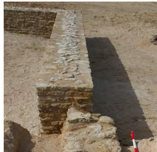
Figure 7.19: Detail of the double-shell masonry of the reconstructed wall. (BF-1051)
