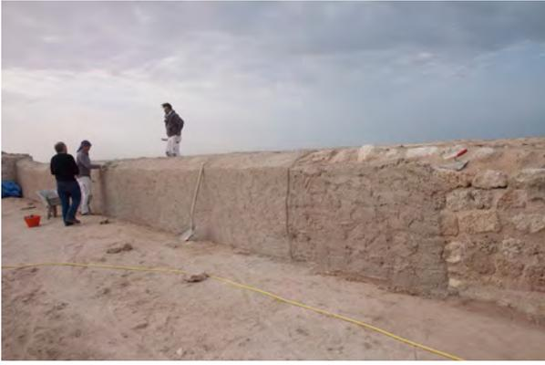
Figure 5.10: Application of the make-up in two layers. (DE-1634)
