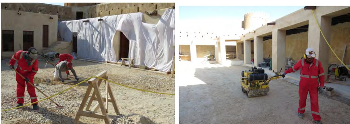
Figure 6.7: Applying the two layers of the new courtyard surface. (ZUTE-0327 and ZUTE-0356)
