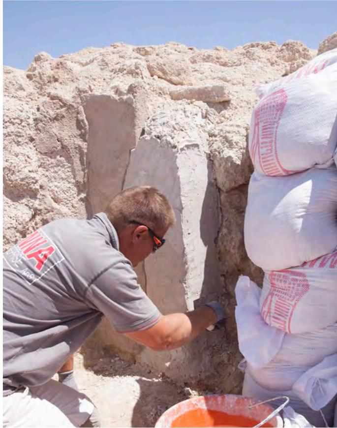
Figure 3.23: Reconstructing the plaster surface on the door jamb, scratching the surface with a knife. (DF-1085)
