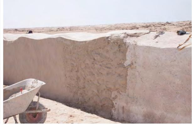
Figure 5.11: Application of the finish plaster layer on the town wall. (DF-0307)
