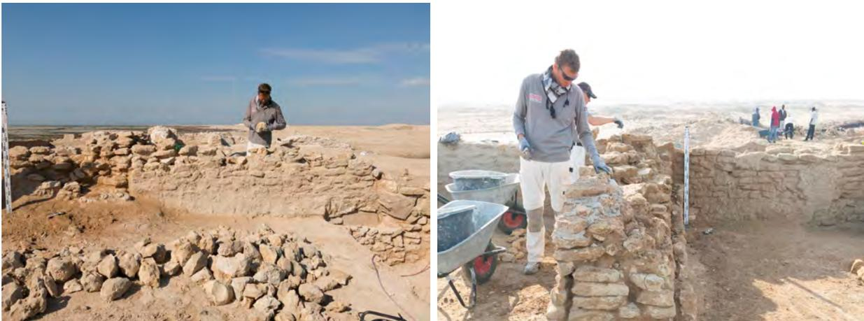
Figure 7.15: Voids in the structure and the capping were closed with dolomite stones and lime mortar. (WE-0100 & WE-0116)
