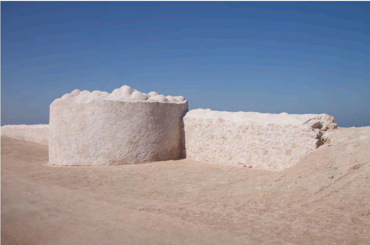
Figure 5.8: T16 after finished consolidation. The rough capping allows better drainage (DF-1076)
