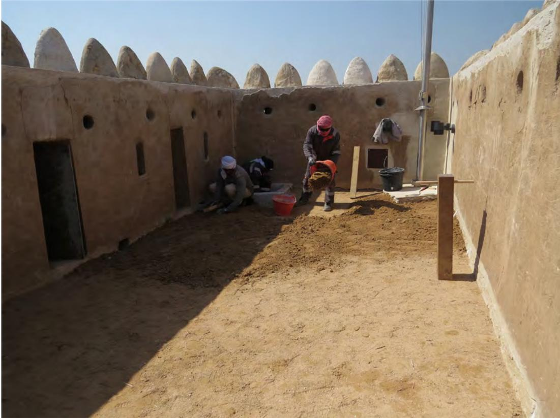
Figure 6.5: Earthen roof on the rectangular tower renewed with traditional techniques. (ZUTF-0568)
