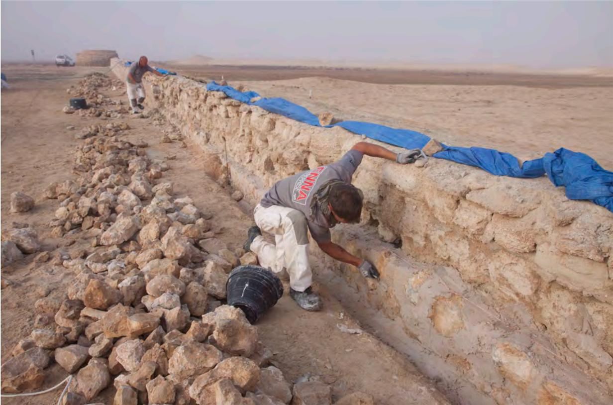
Figure 5.7: The new shell of the Outer Town Wall being constructed in front of the 1980s shell. (DE-0640)
