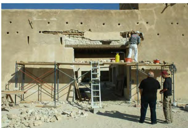
Figure 6.3: Exposed dhow mast above the main gate in October 2013. (ZUUE-0363)
