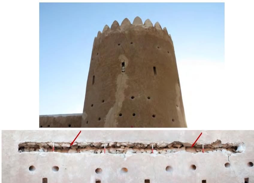
Figure 6.8: View of the south-western tower (top) and a rectified image of the opened interior wall with battlements partially revealed. (ZUTF-2120 and KE-0122)
