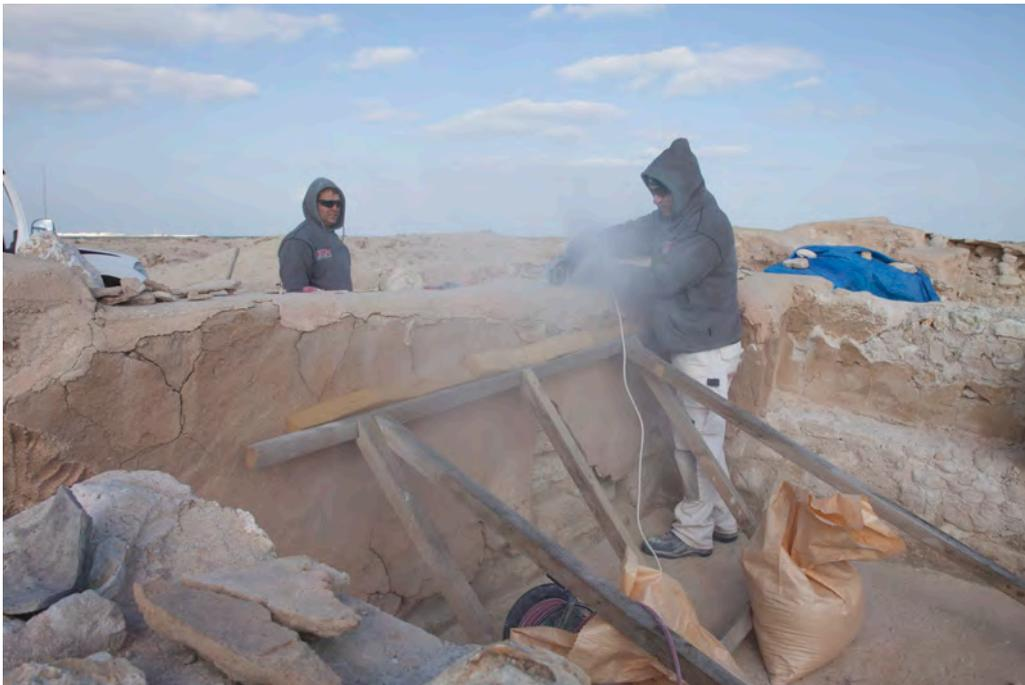
Figure 4.10: Removal of the cement capping on a wall in Space 10006. (DF-0075)
