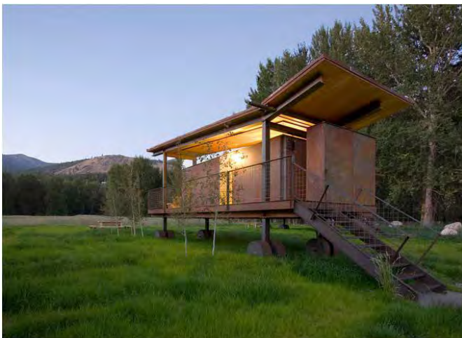
Rollig Huts, Mazama, Washington, USA OSKA Architects Kilde: www.rollighuts.com
